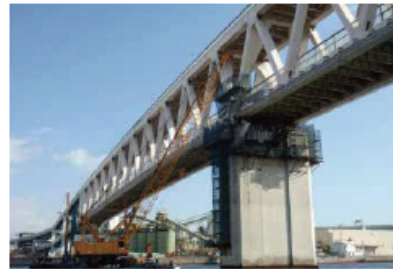
Maintenance work on a bridge
