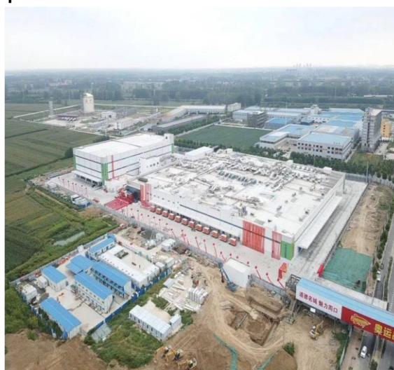
Figure 11: Wilmar's production plant for ready-to-eat food under construction in Henan province
