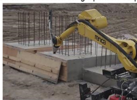
RENCA On-site construction using a portable 3D printer
