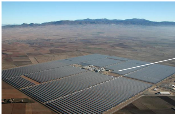
Figure 7. Andasol Concentrated Solar Power Station in Spain (100MWe heat storage 2,000MWh)
