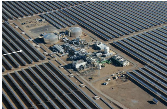
Figure 7. Andasol Concentrated Solar Power Station in Spain (100MWe heat storage 2,000MWh)
