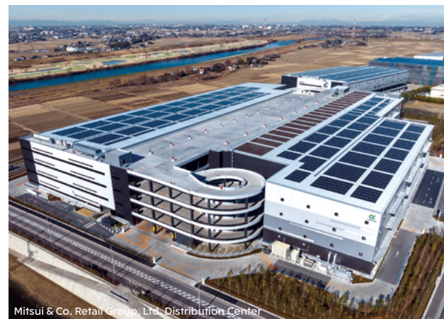
Mitsui & Co. Retail Group, Ltd. Distribution Center
