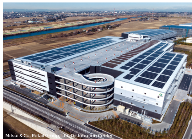
Mitsui & Co. Retail Group, Ltd. Distribution Center
