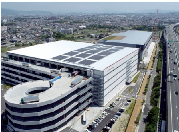
Mitsui & Co. Retail Group, Ltd. Distribution Center
