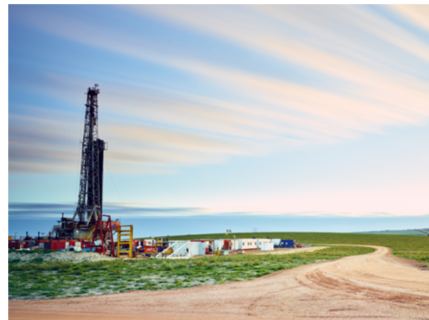
Waitsia Gas Project
