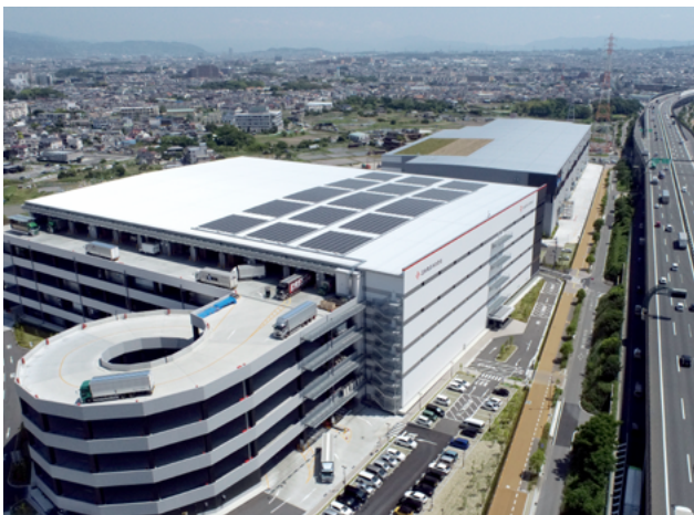
Mitsui & Co. Retail Group, Ltd. Distribution Center
