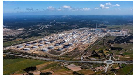
Galp's Sines refinery site for installation of new production facility
