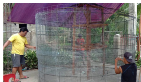
A rainwater storage tank (November 2019)
