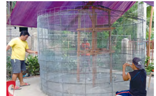
A rainwater storage tank (November 2019)
