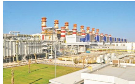
The Ras Laffan C water desalination plant
