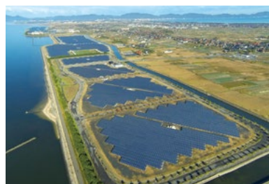
Solar Power Generation Business (Tottori Yonago Solar Park)
