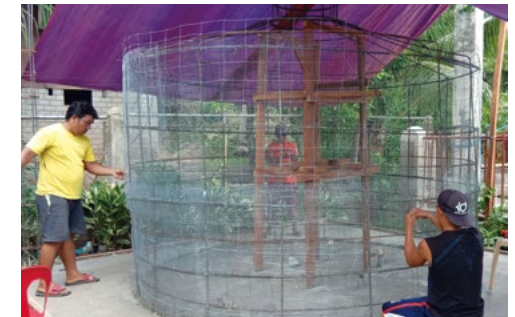
A rainwater storage tank (November 2019)
