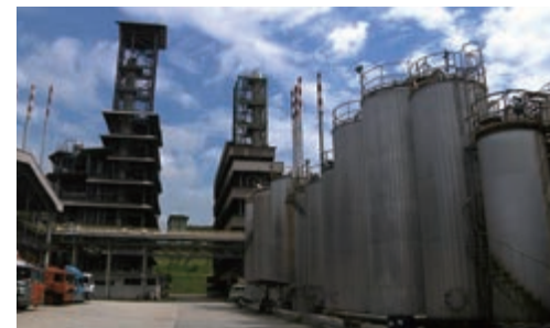
Factory of the oleochemicals manufacturing company
