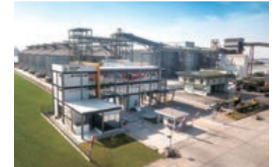
FKSFA's grain import facility
