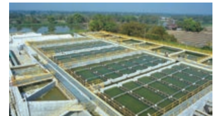
TTW's water purification plant
