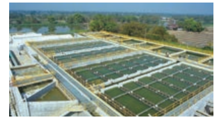
TTW's water purification plant
