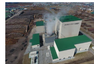
The biomass power station in Tomakomai, Hokkaido
