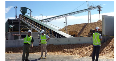
Woodchip processing plant (Bunbury Port in Western Australia)
