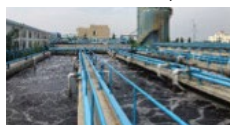
A wastewater treatment facility for purifying factory waste generated in the fruit cleaning process, etc.
