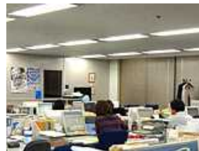
Workspace with high-efficiency lighting and motion sensors installed
