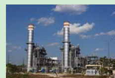
Combined Cycle Valladolid III Power Station, which is operated and managed ecologically
