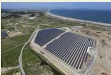
The Mega – solar power generation plant in Higashimatsushima city
