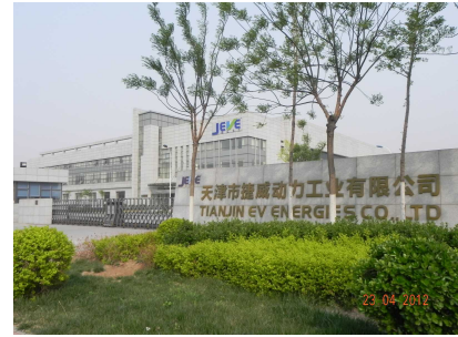
Tianjin EV Energies factory construction
