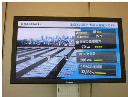
Power savings are visible on a display in the lobby
