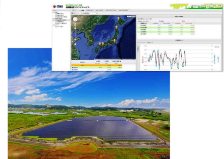
Conceptual image of solar power generation facilities and a remote monitoring screen
