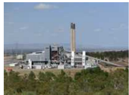
Oxyfuel combustion boiler at the Australia Callide-A coal-fired power station in Queensland, Australia
