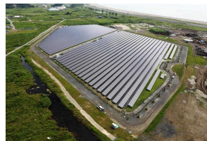
Okumatsushima “Kizuna” Solar Park (Higashimatsushima City reconstruction project)
