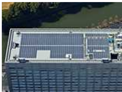
Solar panels installed on the roof of the head office building
