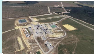
Waitsia Gas Field (Under development)
