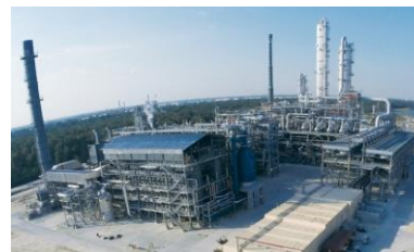
Fairway (US) methanol plant (Annual capacity of 1.3m tons; Mitsui has 50% stake)
