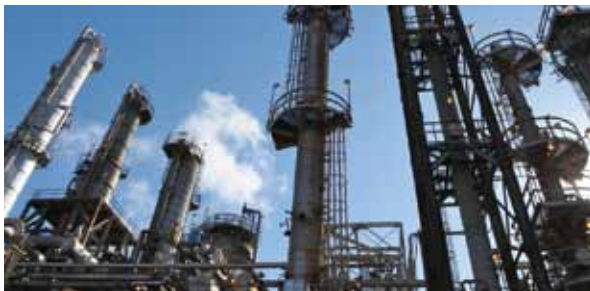
Celanese methanol derivative (ethanol) plant
