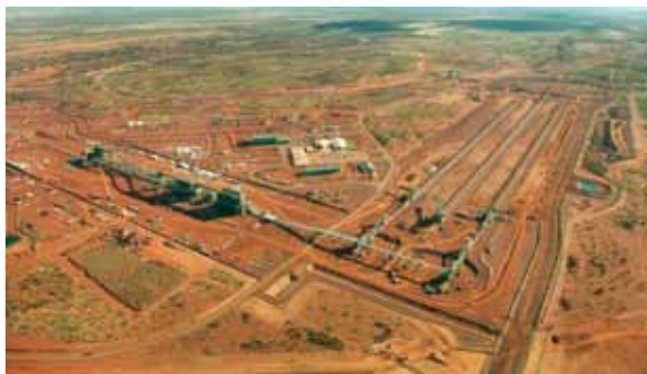
Iron ore processing equipment and stock yard at Jimblebar iron ore mine, currently under development (source: BHP Billiton)
