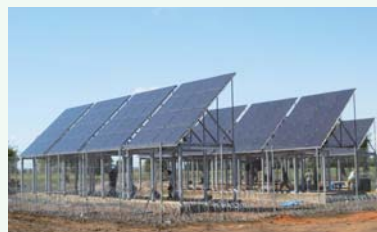
A solar-powered irrigation facility under construction
