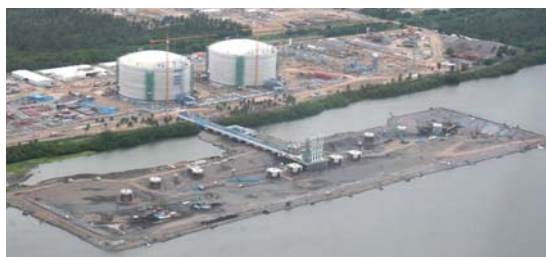
Manzanillo LNG terminal, currently under construction
