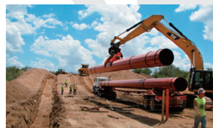
Pipeline laying operation site
