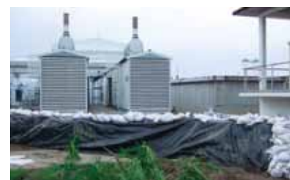
A levee built to prevent flood water from reaching the water treatment facility
