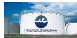
US : tank terminal for chemical products
