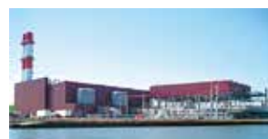
IPP(US : Astoria I gas power plant)
