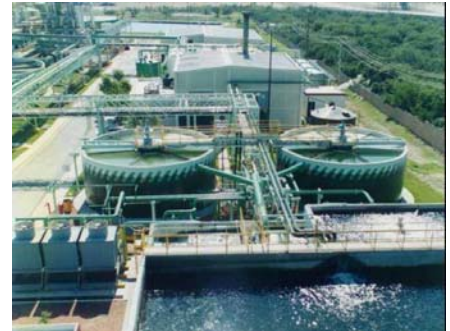
Atlatec waste water treatment plant in Mexico
