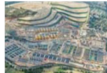
Water Treatment (Atotonilco)
