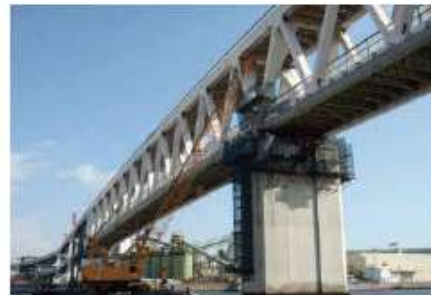
Maintenance work on a bridge
