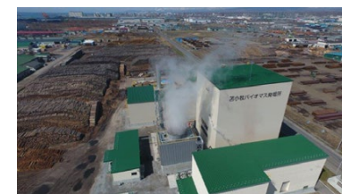
Tomakomai Biomass Power
