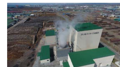
Tomakomai Biomass Power
