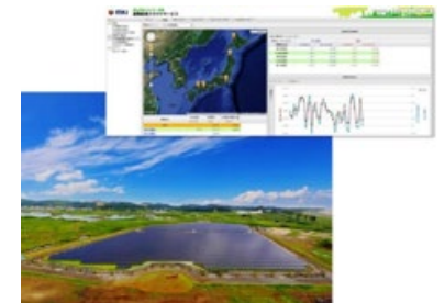
Conceptual image of solar power generation facilities and a remote monitoring screen
