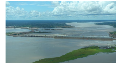
An aerial view of the power plant
