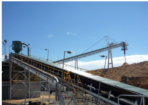
Woodchip processing plant (Bunbury Port in Western Australia)
