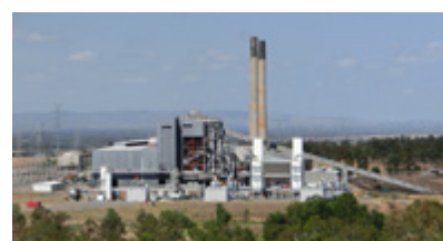
Oxyfuel combustion boiler at the Australia Callide-A coal-fired power station in Queensland, Australia
