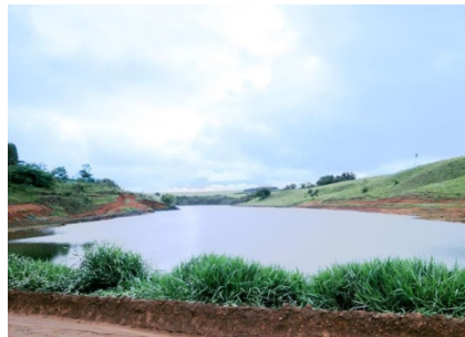
An extended dam to secure irrigation water
