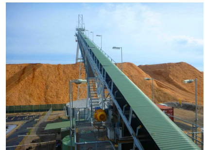
Woodchip production plant (Bunbury Harbour in Western Australia)
