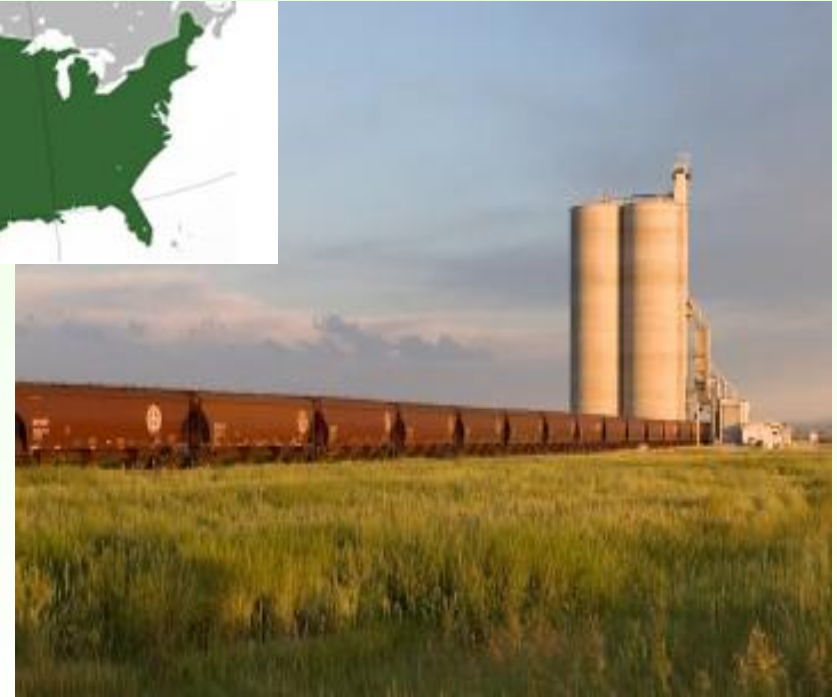
UGC's grain country elevator in Montana, U.S.
