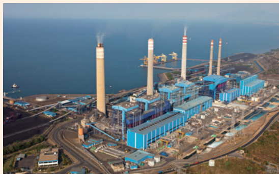
Paiton coal-fired thermal power plants (Paiton 1 (foreground) and Paiton 3 (third from front))
