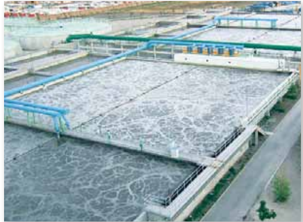
EL AHOGADO wastewater treatment plant
