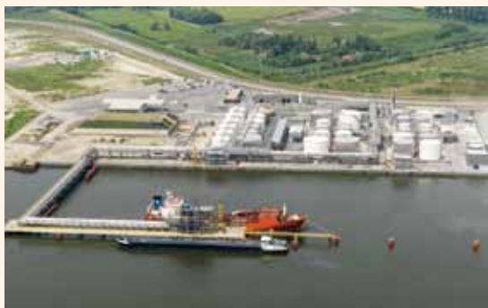
ITC Rubis tank terminal
