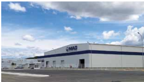
MAG's Steel Service Center
