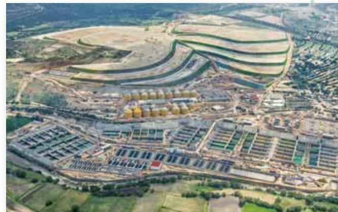
Atotonilco wastewater treatment plant (under construction)
