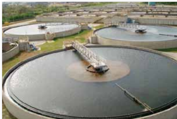
Wastewater treatment plant in Trinidad and Tobago
