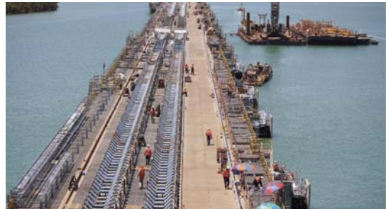
The Port Headland facility under expansion project
