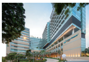
④Mount Elizabeth Novena Hospital, an IHH hospital (Singapore)
