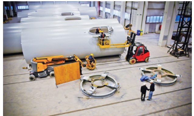
Wind power generation tower under construction
