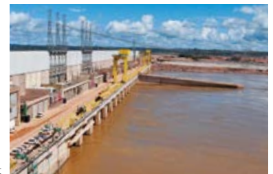
Jirau Hydroelectric Power Plant
