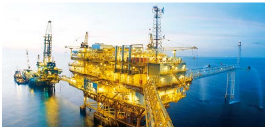
Mitsui Oil Exploration Co., Ltd., Gas Production Facility, Gulf of Thailand
