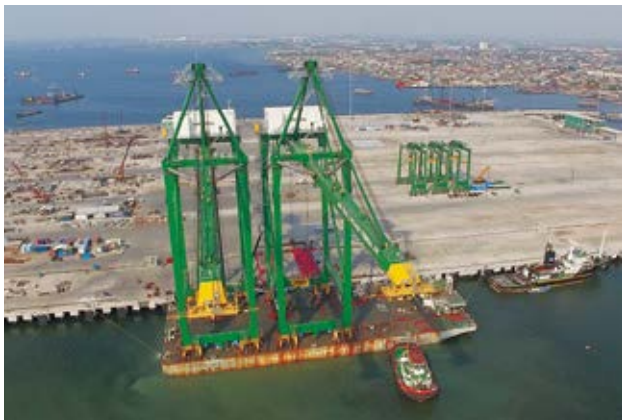
Offshore container terminal at Tanjung Priok Port under construction
