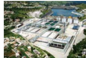
Agua Prieta wastewater treatment plant invested in by subsidiary ATLATEC, S.A. de C.V. (Mexico)
