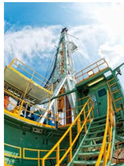
Drilling rig at Marcellus shale gas project (US) ©Anadarko Petroleum Corporation
