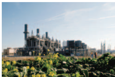
The combined-cycle power plant in Ontario, Canada
