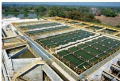
Water supply project of Thai Tap Water BOO, Thailand
