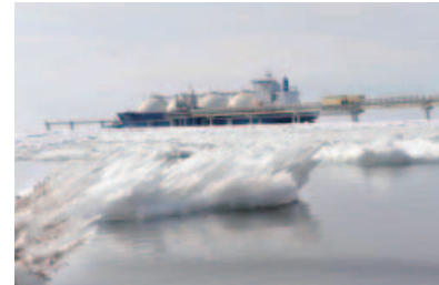
The Sakhalin II project, Russia ©Sakhalin Energy Investment Company Ltd.
